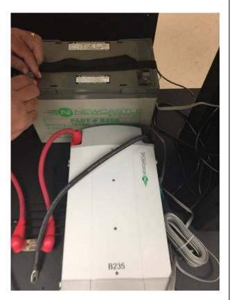
**2.** Carefully place battery on base and strap down as shown above.
