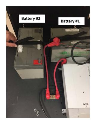
**2.** Carefully place batteries on base (as shown above) and securely tighten straps.
