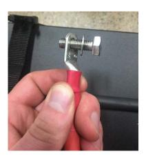
**7. Positive Connection, Battery 2:** Take bolt and place flat washer, large red wire (B) onto bolt (as shown above); insert bolt into positive (+) battery terminal.
