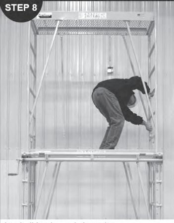
Attach all four braces before using.
