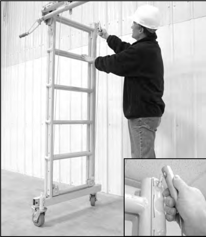
5) Attach cable ends to hooks on top of end sections.
